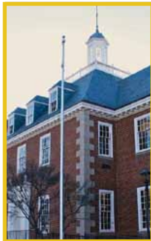
Councilmember Bowser joined Mayor Gray, library officials and community members at a ribbon cutting for a beautiful new Petworth Neighborhood Library which reopened on February 28th after a $12 million, 14-month renovation. Work done on the library includes an updated floor plan, restored windows and doors, a repaired roof, improved ADA access, a new elevator, electrical and fire alarm upgrades, a new outdoor activity area and a 100-person meeting room, among other additions.
